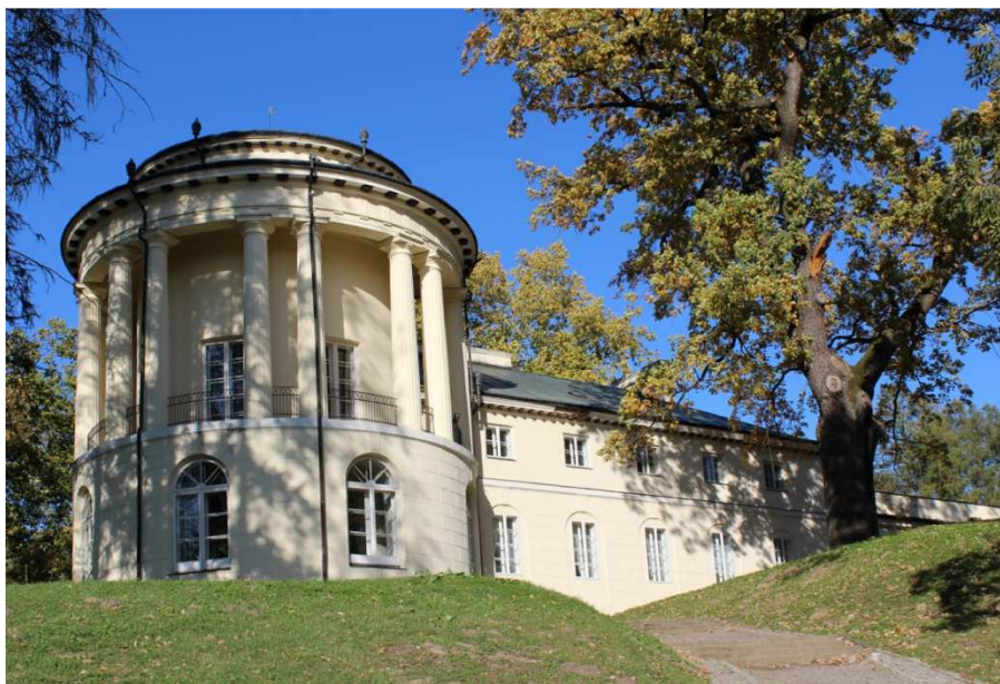
Figure. 1. The palace in Zarzecze – general view
