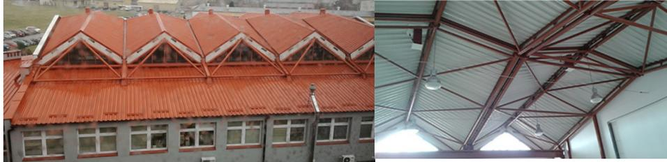
Fig. 1. A roof composed of repetitive shell segments and its structural system:
