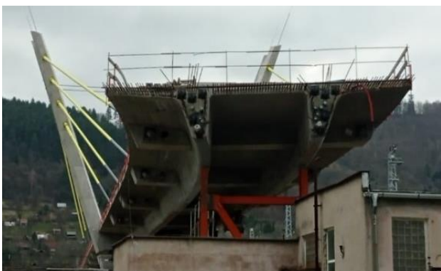
Fig. 3. Box girder bridge: extradosed bridge in Zilina
