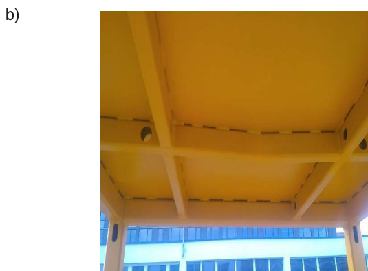
Fig. 15. FOPS structure under test procedure (a) and roof deformation after impact load (b)
